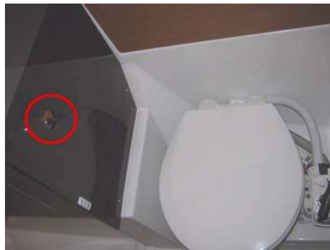
Drainage pump control - Shower
