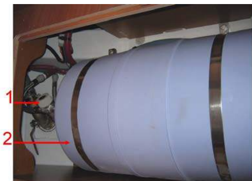
Water heater 220V- Saloon seating Starboard
