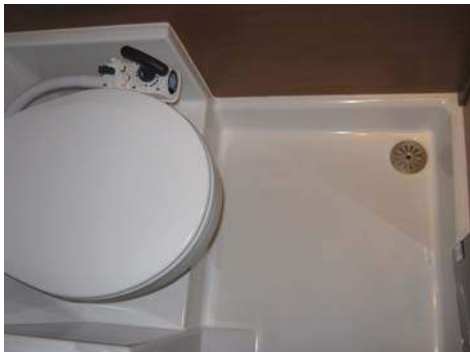
Drain plug - Shower draining
