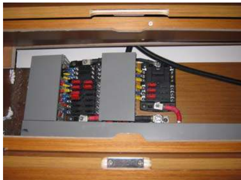
Fuse board - Back of electrical panel
